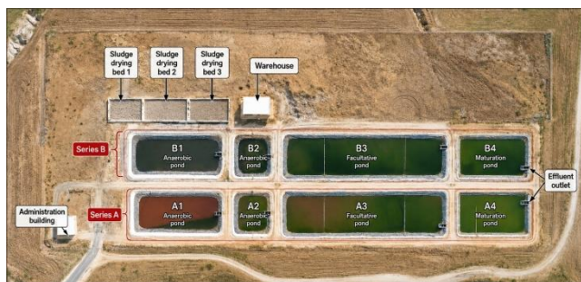
Figure 1. Annotated aerial view of the Fayda WSPs.
